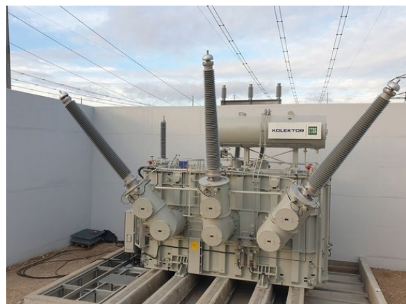
Figure 5 – 400kV Transformer
