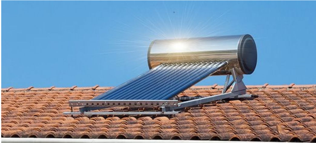
Figure 6- Solar Thermal Panels
